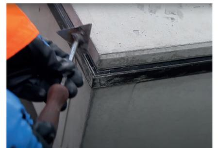
After concreting & deforming of the tunnel segment the flawless fit of the gasket has to be checked. In case that concrete slum has penetrated to the gaskets sides and surface it should be removed.
