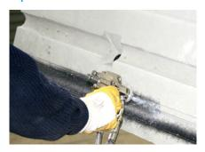
The adhesive has to be applied with a Spraygun which is specially designed to apply the SEALABLE adhesive in the form of "hairs". The spraying process should not take more than 5 minutes for one segment. It is important that the adhesive is evenly applied into the groove bottom and onto the side walls. The side walls are the main contact area for the bondingprocess.
