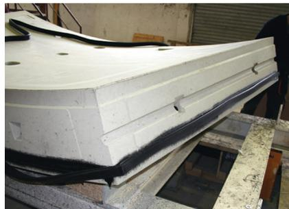
Two workers should start with placing the corners and short gasket sides into the groove simultaneously. The process should be started with the correct positioning of the corners and pressing the gasket into the groove by hand.
