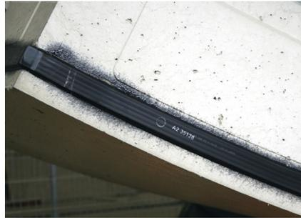
During the final control each gasket corner position should be double checked. The gasket corner should be in line with the segment corner. As well the correct type of gasket and positioning of the complete gasket in the groove should be checked. After 72 hours the adhesive will achieve its final strength, after this time the adhesive bonding should be checked visually.
