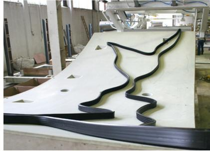
The gasket has to be installed after the adhesive is “tacky”. The installation should be done by two workers. They should place themselves opposite on each of the short sides of the segment.
