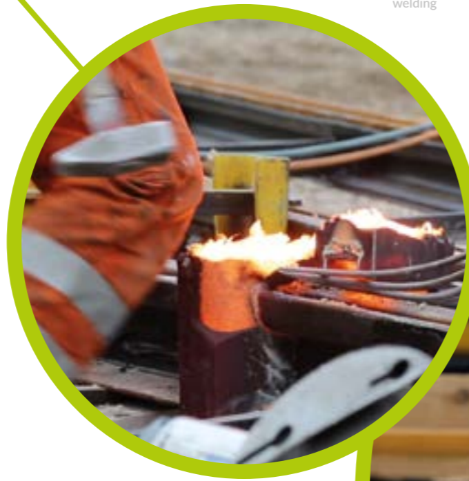
Joint welding of the rails by means of thermite welding
